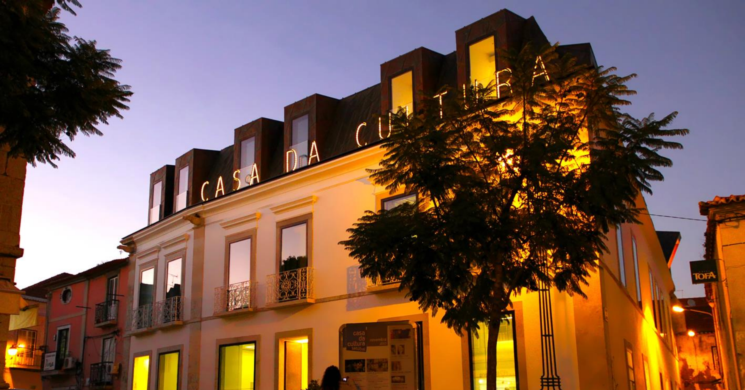
INSTALLATION OF CASA DA CULTURA (HOUSE OF CULTURE)
