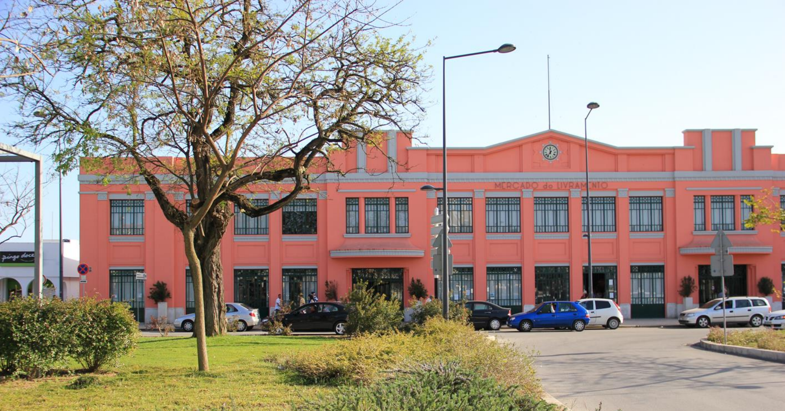
UPGRADING AND MODERNIZATION OF THE MERCADO DO LIVRAMENTO (MARKET)
