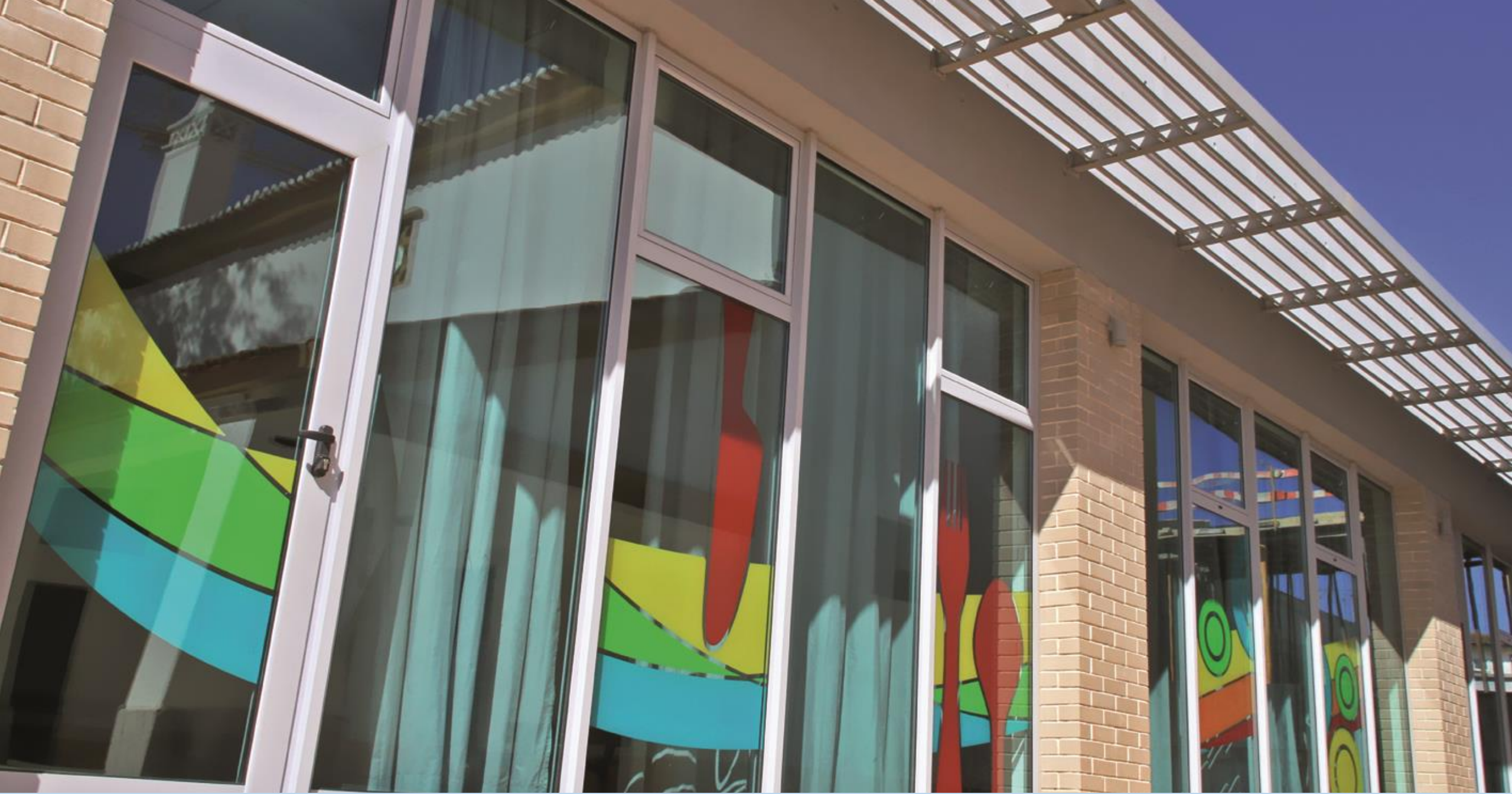
AFONSO COSTA ELEMENTARY SCHOOL
