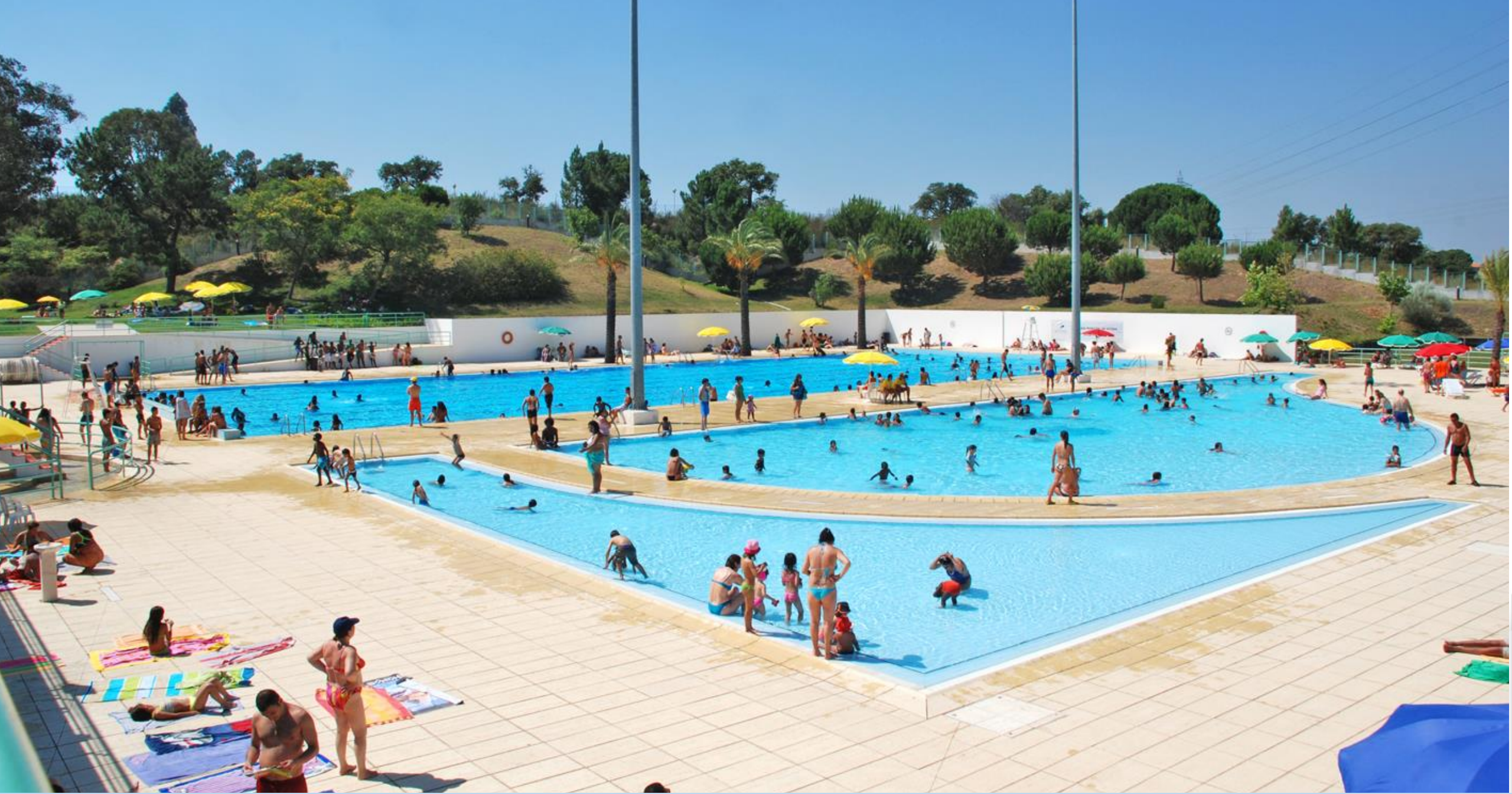
RENOVATION AND IMPROVEMENT OF THE MUNICIPAL SWIMMING POOL COMPLEX
