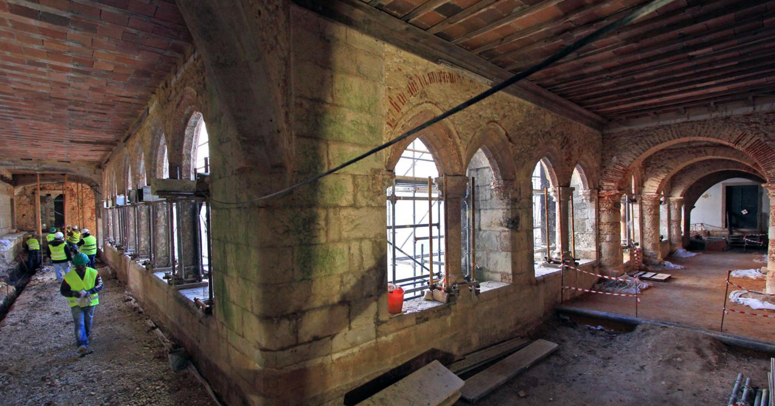
RECOVERY AND ENHANCEMENT OF CONVENTO DE JESUS (CONVENT)
