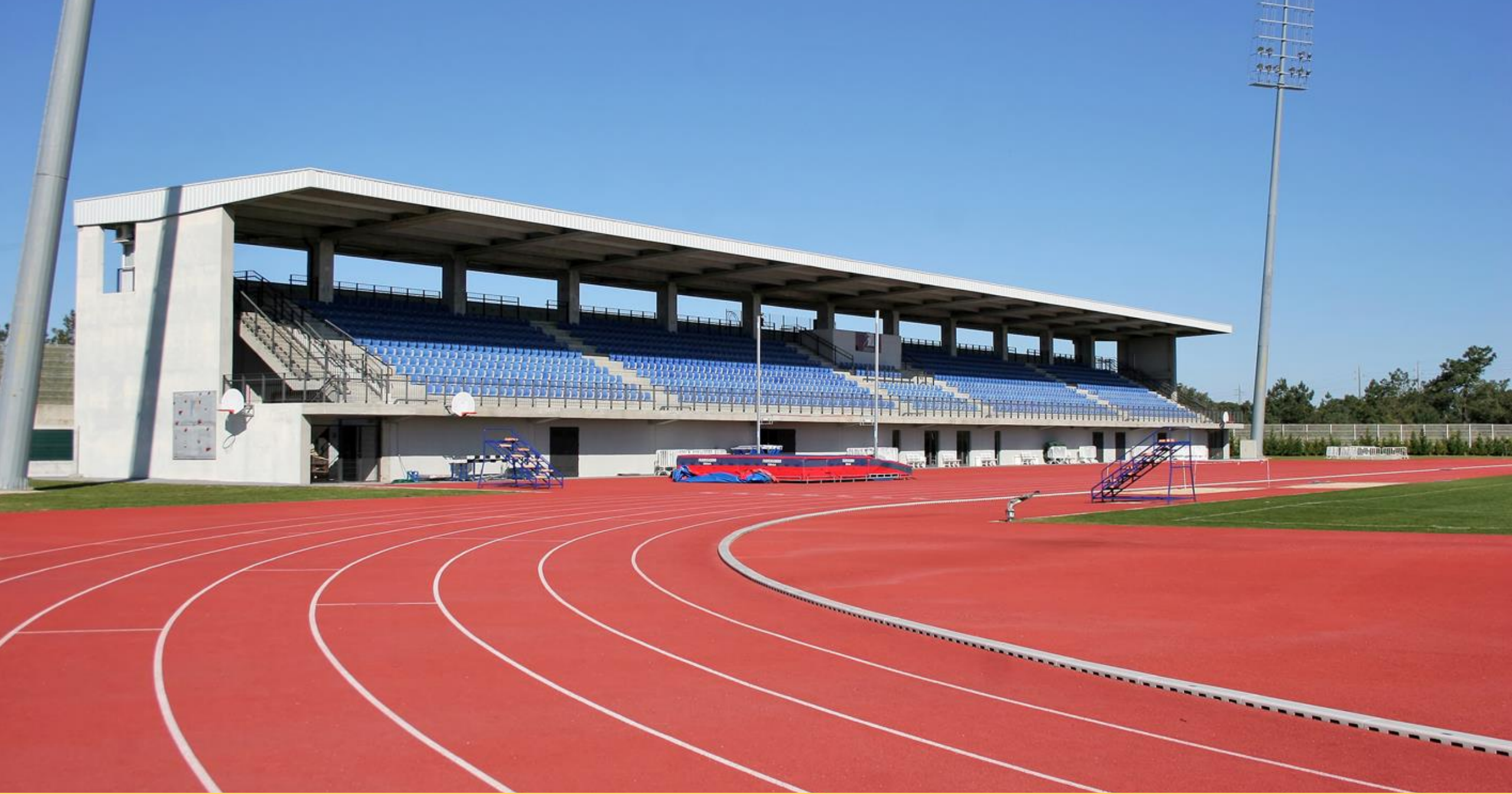
CONSTRUCTION OF AN ATHLETICS TRACK
